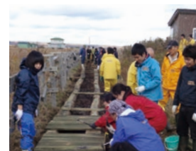
The wooden walkway repairs that took place in 2013
