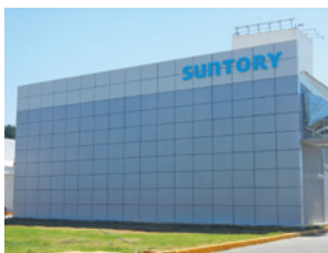
New utility building
