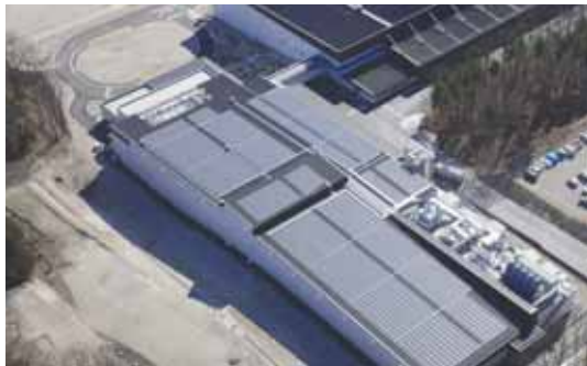
▲ Solar panel at Minami Alps Water Plant of Suntory Products Ltd.
