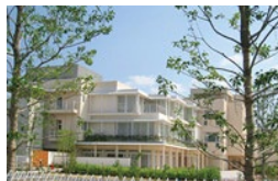
Domyoji-Takadonoen, a general-purpose welfare facility
