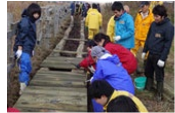
Landscape repair of boardwalk (2014)
