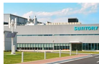
Suntory Products Ltd. Kanagawa Ayase Plant uses rainwater to water plants
