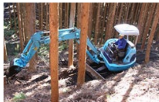
Road making with low environmental impact
