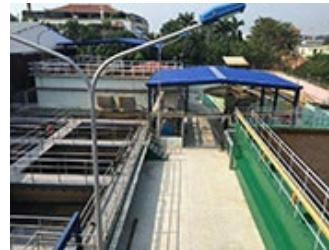
Waste water treatment plant
