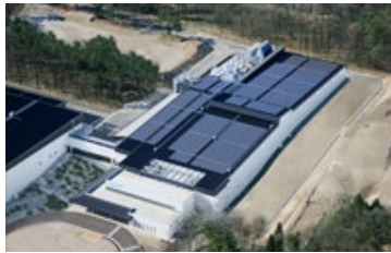
The Minami Alps Hakushu Water Plant of Suntory Products Ltd.
