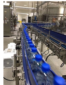
Newly installed water line in PBV's Winston-Salem production facility
