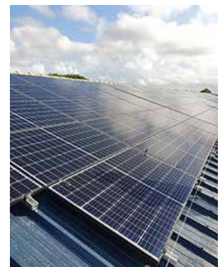
New solar panels installed on the roofs of the fermentation facility
