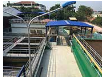
Waste water treatment plant
