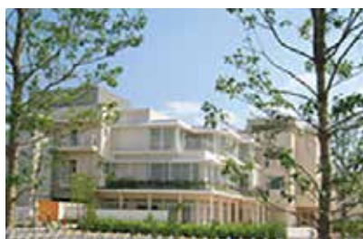
Domyoji-Takadonoen, a general-purpose welfare facility
