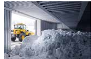
Snow room at Okudaisen Bunanomori Water Plant of Suntory Products Ltd.
